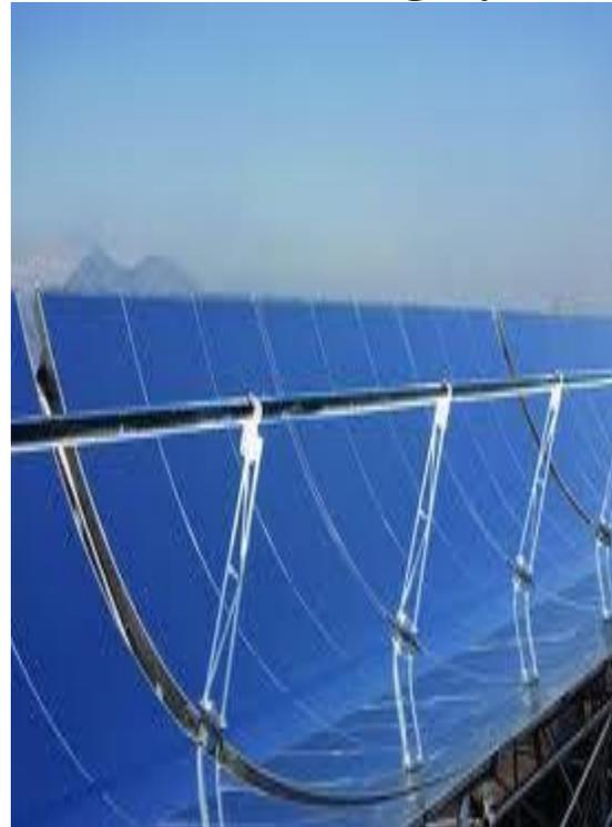
Although many solar technologies have been demonstrated, parabolic trough solar thermal electric power plant technology proves to be one of the major renewable energy success stories of the last two decades. Among all the solar energy systems, parabolic troughs are one of the lowest cost solar electric power options available today and have significant potential for further cost reduction.
