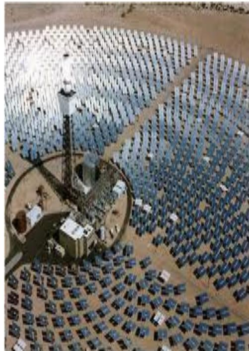
It is also known as a power tower. It is a solar power facility that uses a field of two-axis tracking mirrors known as heliostats (devices that track the movement of the sun). Each heliostat is individually positioned by a computer control system to reflect the sun's rays to a tower-mounted thermal receiver. The effect of many heliostats reflecting to a common point creates the combined energy of many suns, which produces high
