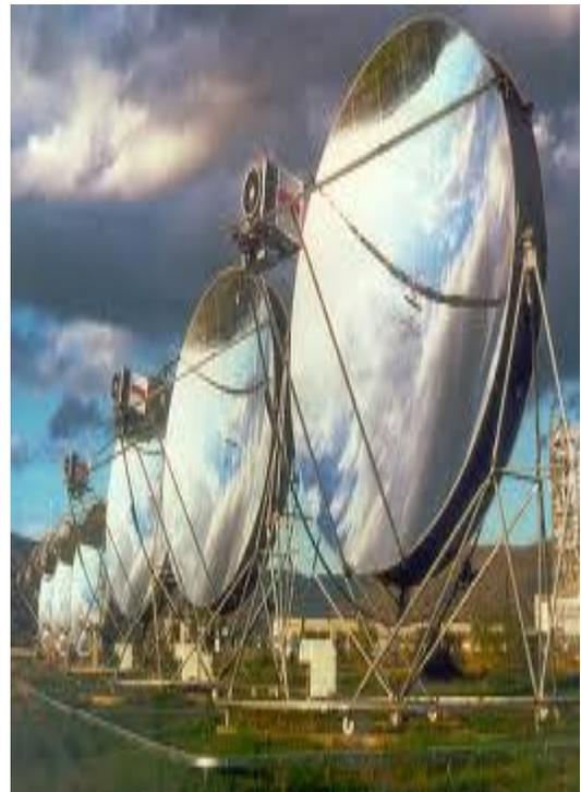
The dish or Stirling system generates power by using parabolically arranged mirrors to reflect sunlight onto a small focal receiver, thereby heating a gas chamber connected to a piston and drive shaft. The drive shaft powers a generator which produces electricity to be distributed to a grid.
