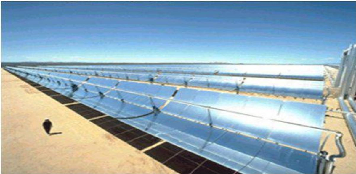
Computer systems manage the mirror positions, tracking the motion of the sun throughout the day to maintain the focus point on the absorber. At night and during stormy weather, the reflector units invert, exposing steel to the sky for maximal resistance to weather events such as ice, hail and high winds.
