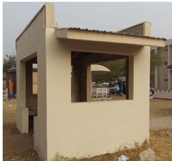
Figure 1: A Gazebo built with Ashment:OPS concrete.
